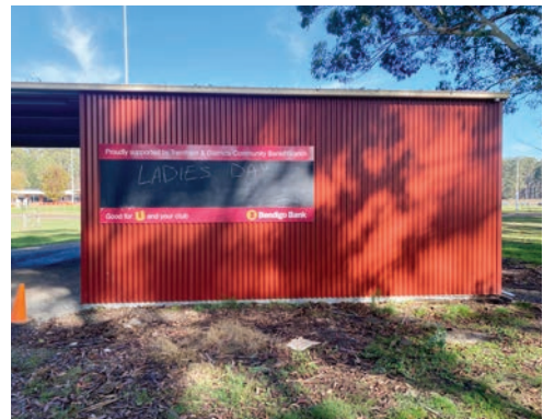
Trentham Sports Ground Gatehouse
